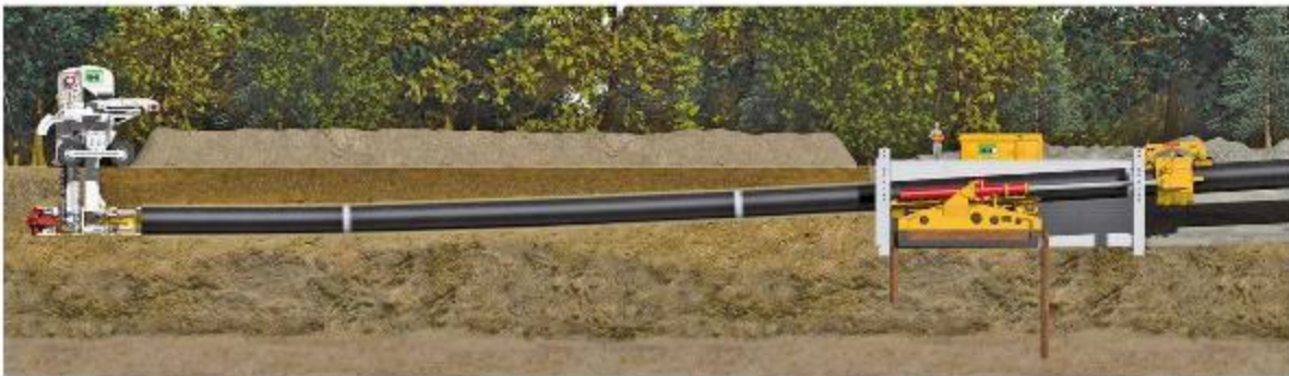
The push force delivered by Herrenknecht Pipe Thruster.
